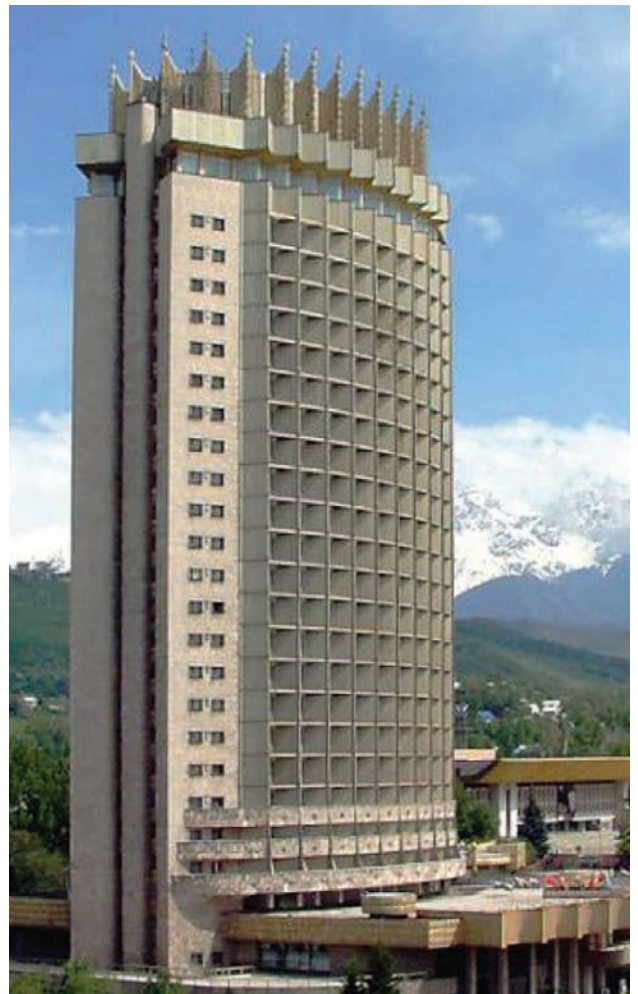
Fig. 25. Yu. Ratushny and others. Hotel "Kazakhstan" in Alma-Ata, 1978. Source: Ruslan Muradov archive
