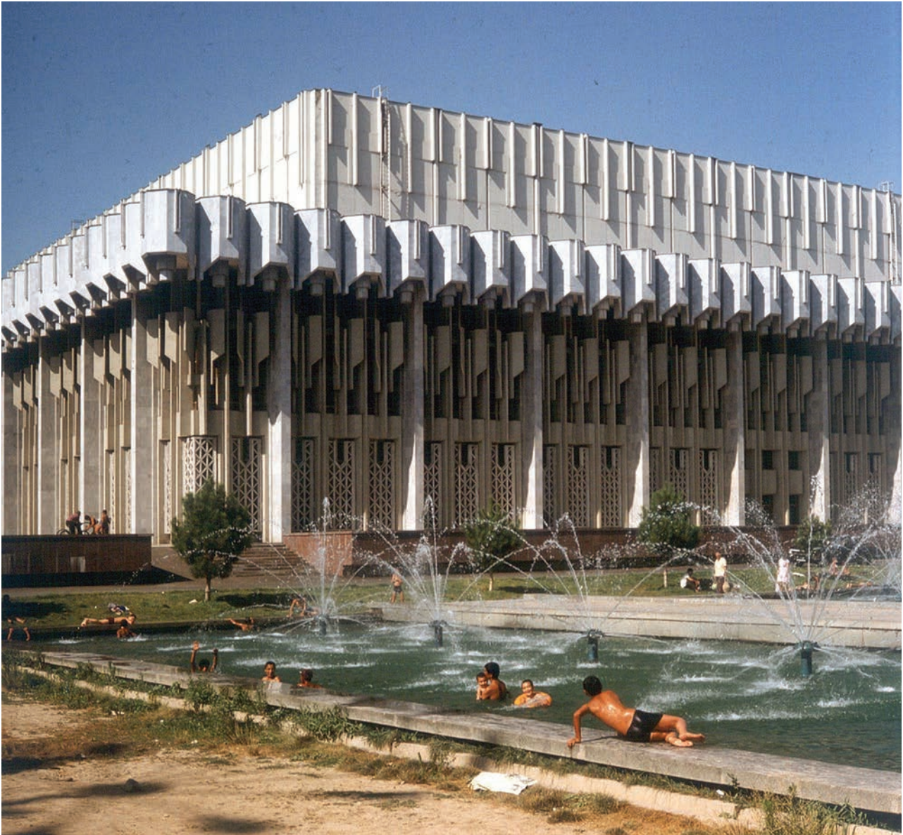
Fig. 30. E. Rozanov et al. Palace of Friendship of the Peoples in Tashkent. 1982. Photo: Werner Starke. Source: postvu.com/717649
