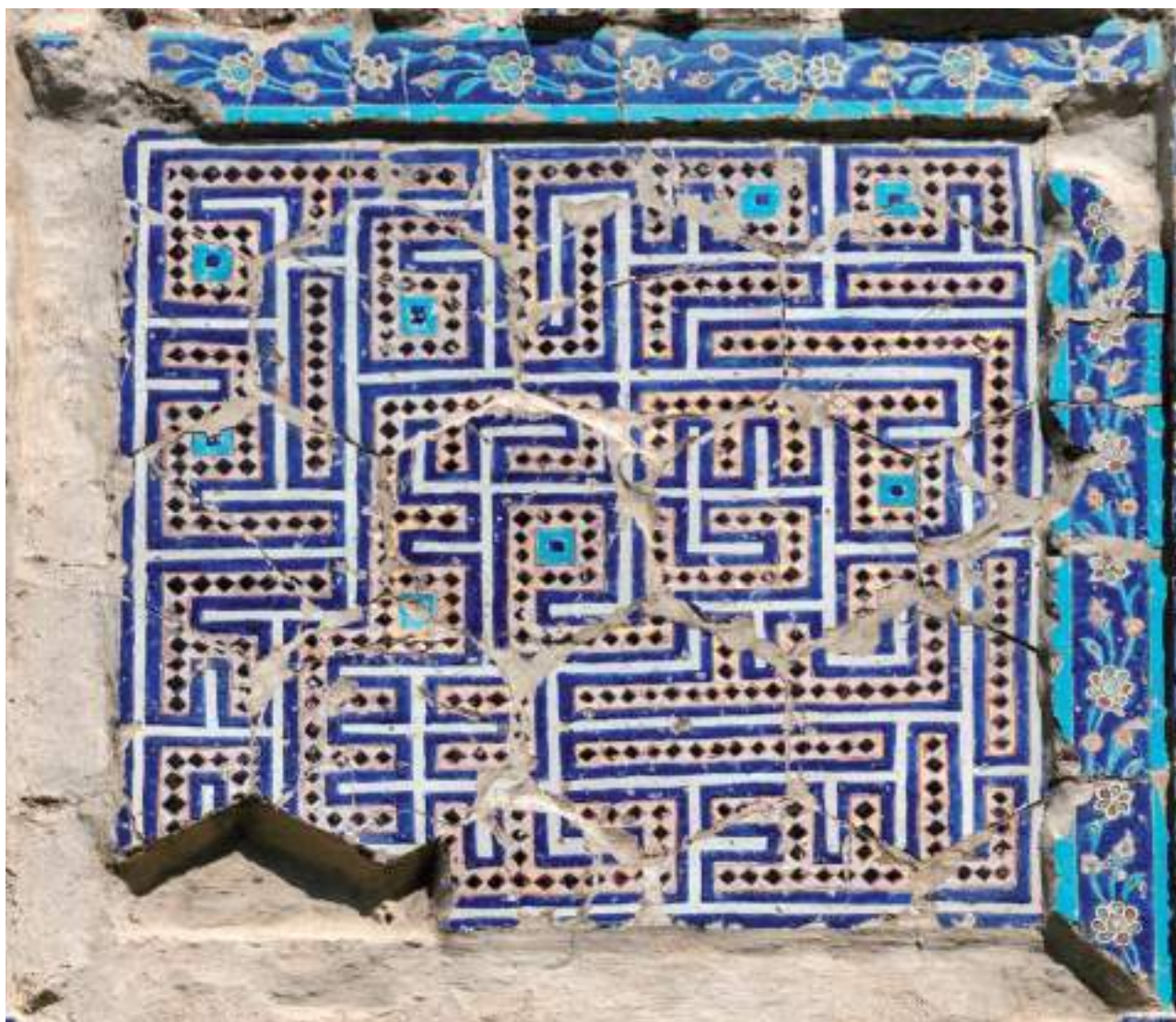
Fig.12. Shahr-i Sabz, Aq Saray palace (1379-96), detail of cuerda seca tiles on entrance (photo: B. O'Kane).
