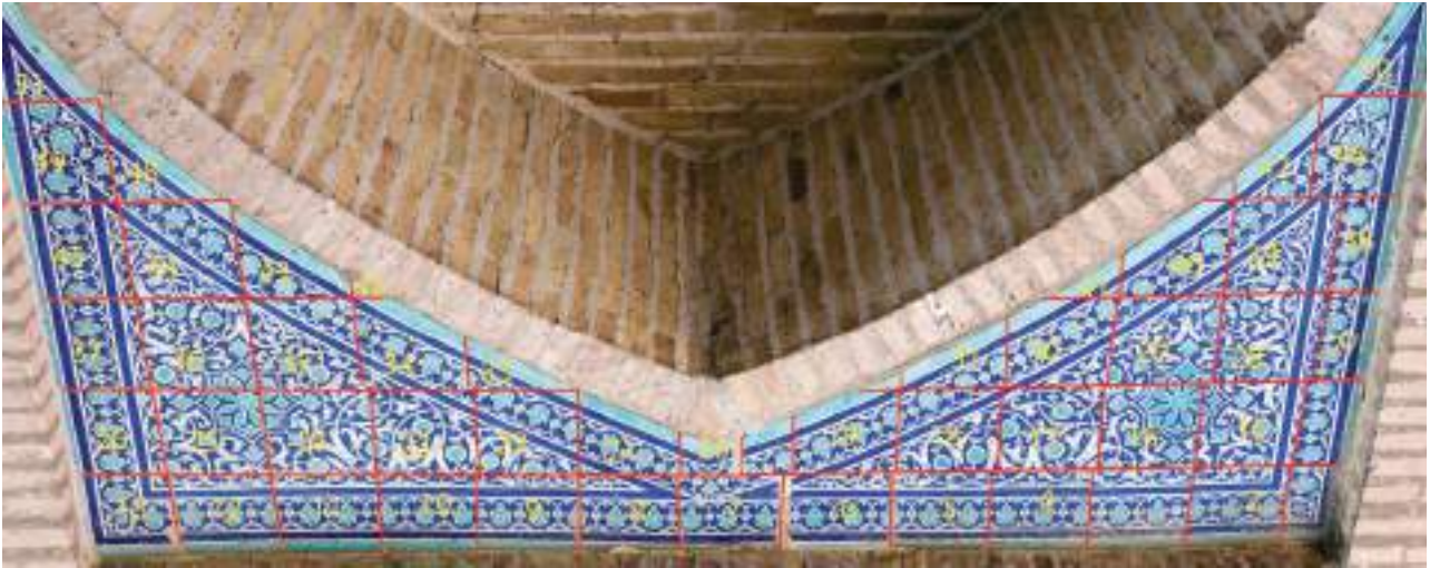
Fig.23. Khiva, Muhammad Amin Khan madrasa (1851-5), spandrel (photo: B. O'Kane). Red lines added to show tile divisions.
