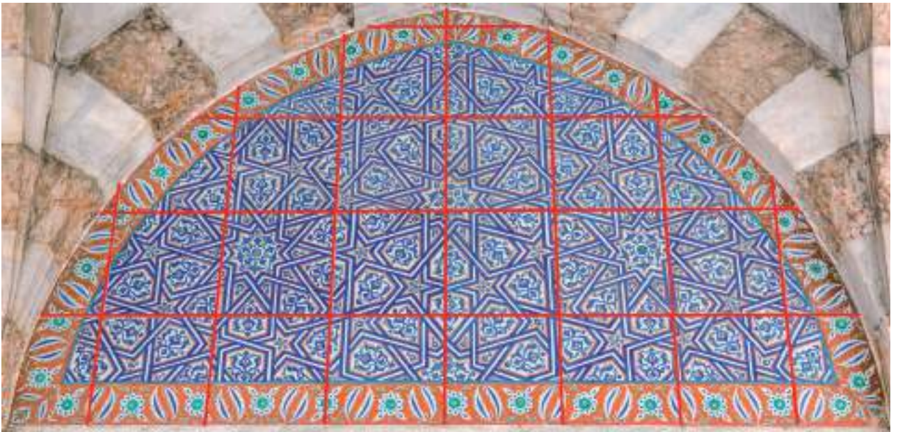
Fig.26. Istanbul, Hagia Sophia, mausoleum of Sultan Selim II (1577), tympanum above entrance (photo: B. O’Kane). Red lines added to show tile divisions.
