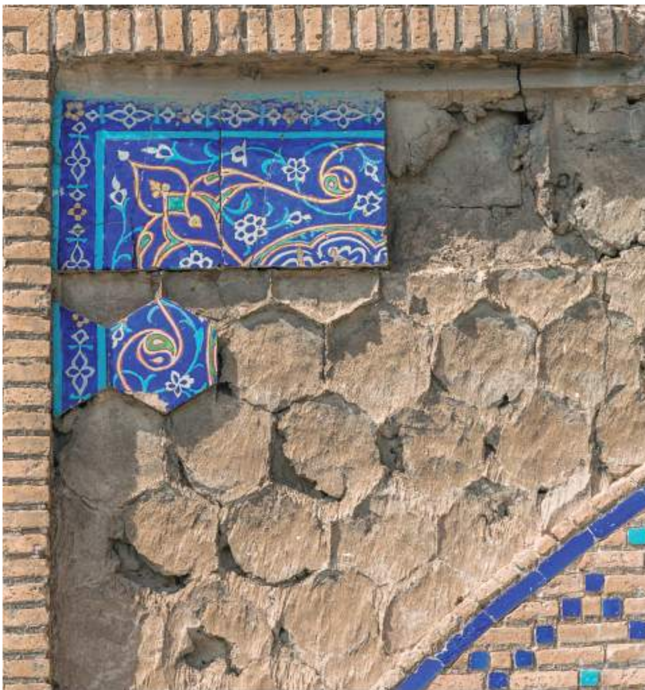
Fig.11. Samarqand, Bibi Khanum mosque (1399-1404)), detail of cuerda seca tiles at side of entrance ayvan (photo: B. O'Kane).
