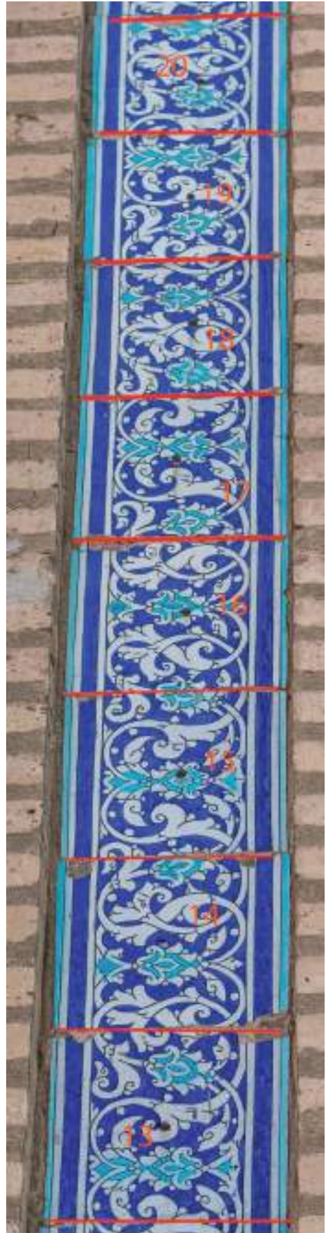
Fig.20. Khiva, Muhammad Amin Khan madrasa (1851-5), panel (photo: B. O'Kane). Red lines added to show tile divisions.
