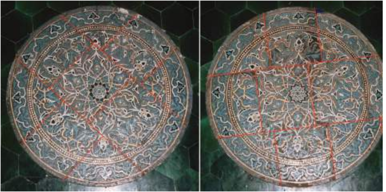
Fig.24. Bursa, Yeşil Cami (1421), detail of cuerda seca dadoes (photos: B. O’Kane). Red lines added to show tile divisions.
