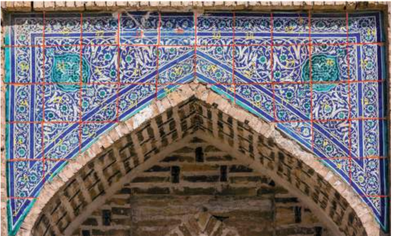
Fig.21. Khiva, Muhammad Rahim Khan madrasa (1871), spandrel (photo: B. O'Kane). Numbers of original tiles marked in yellow; of replacements in orange. Red lines added to show tile divisions.
