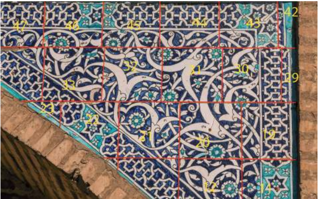
Fig.22. Khiva, Allah Quli Khan madrasa (1834-5), spandrel (photo: B. O'Kane). Red lines added to show tile divisions.
