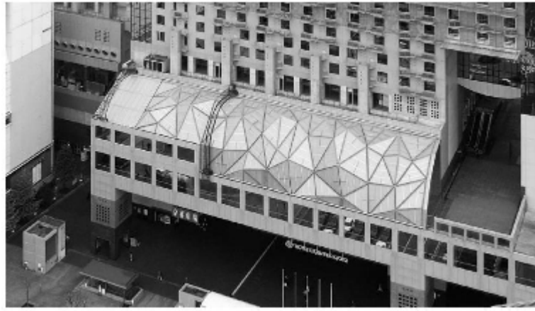
Figure 6. Geometrically complex but topologically uniform cellular surface of a roof. Every triangular surface of the demonstrated buildings has three triangular neighbors
